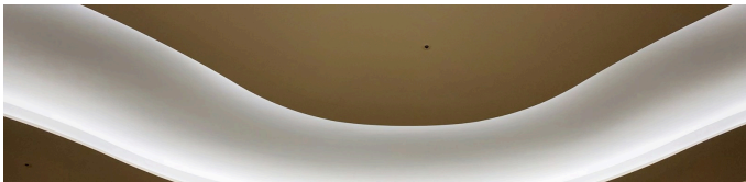
Curved cove: a continuous run follows the plan with no visible pitch and no hot spots at the joins.
